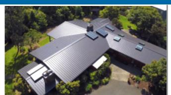
The StreamLine™ Standing Seam is the only metal roofing panel with a patented no-siphon dry lock seam, with a unique reversing feature to allow installation of panels from both directions starting at any location. The panel is designed with softer, less industrial lines to provide an architecturally pleasing appearance.
